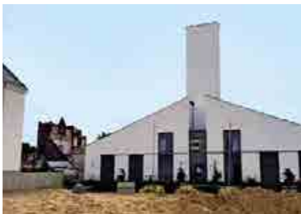
Co-generation plant at the "52 Grad Nord" project in Berlin
